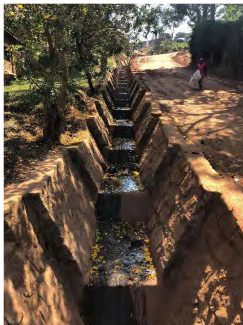
Figure 4.57 Open masonry channel
