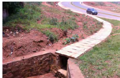
Figure 4.58 Covered masonry channel
