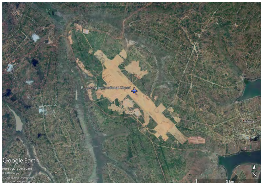
Figure 4.36 Google Earth View of Bugesera International Airport under construction
