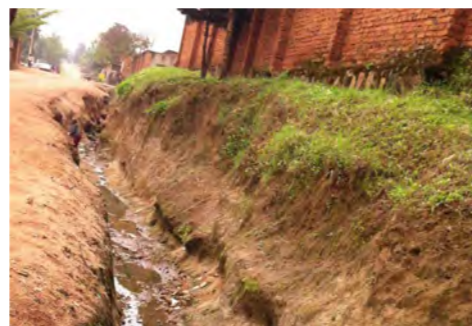
Figure 4.59 Unlined natural channel
